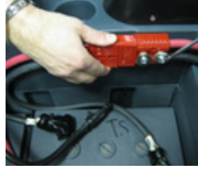
3 Check battery cables are well connected together.
